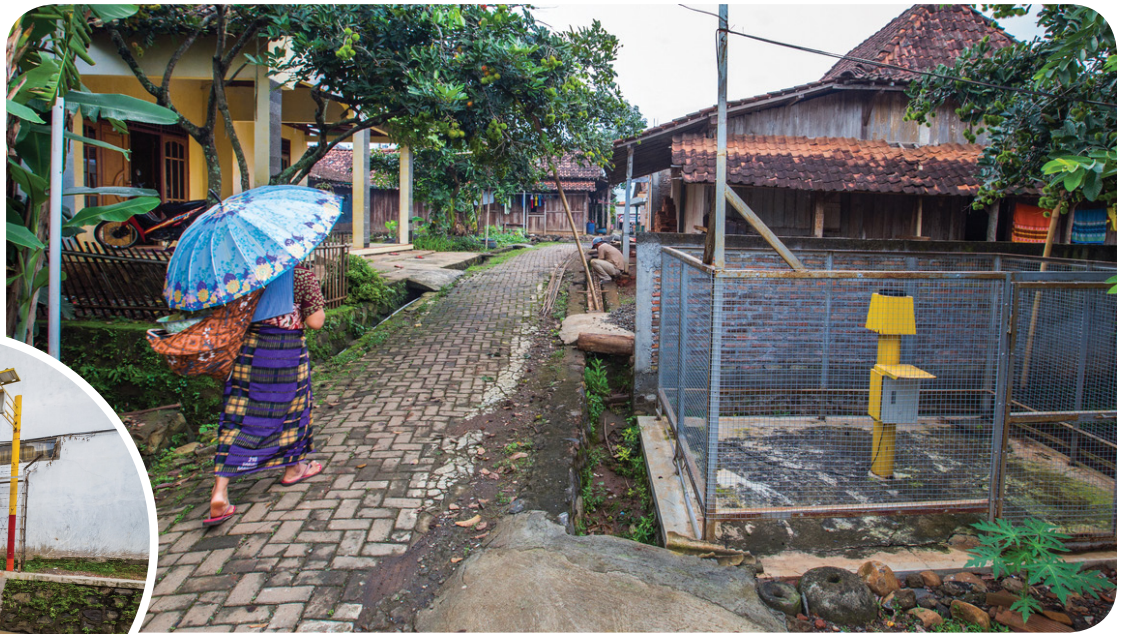
<----- Alat Pencatat Ketinggian Muka Air dipasang di sepanjang DAS Beringin, Semarang. Automatic Water Level Recorder installed along Beringin Watershed, Semarang.
