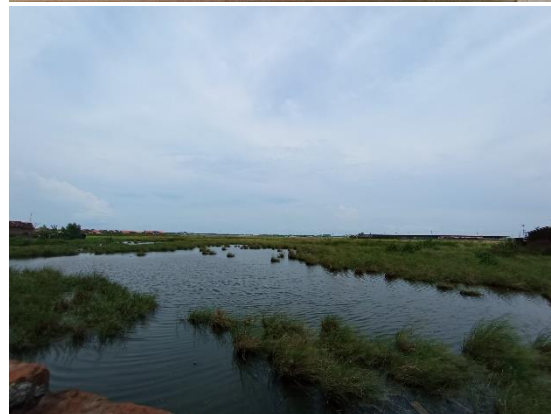
(d) Embankment construction and area that is still flooded in RW 08
